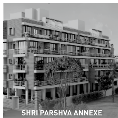
SHRI PARSHVA ANNEXE
